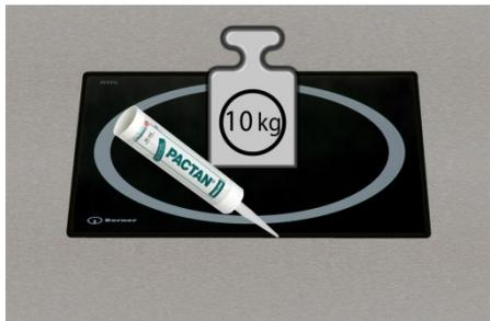
Fill the place between the glass ceramic plate and surface with excess pactan.
