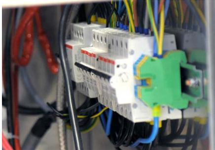
Fasten the fuse and connection rail. Provide an easy access and a splash-proof installation. In case of a fault the fuses need an easy access to turn it on again. It's an additional backup of the system.
